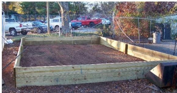
Figure 1—Constructed gravel bed wooden frame.
